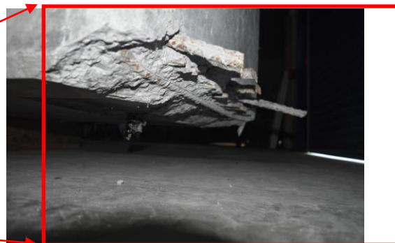
d) Steel reinforcement and concrete condition at the west end of the beam
