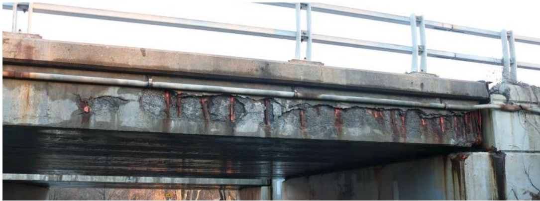
a) Spalled concrete and corroded reinforcement at a fascia beam
