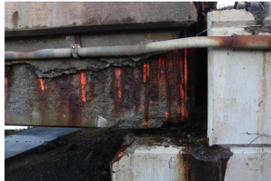
c) damage at the abutment
