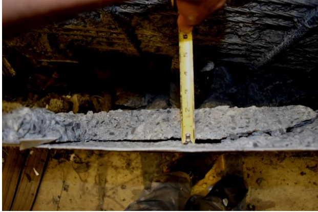
a) spalled concrete cover
