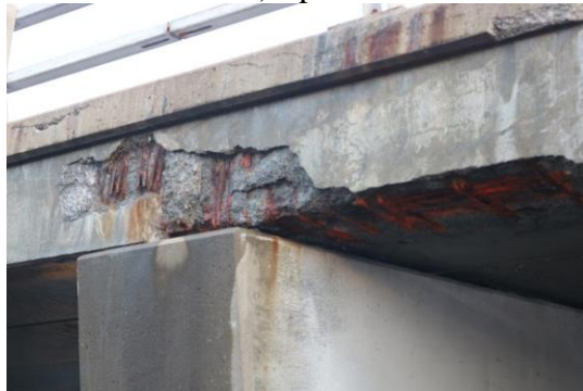
b) damage at the pier support
